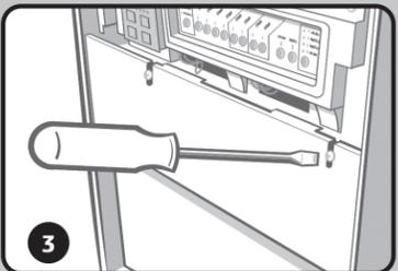
Reinstall the dead panel (close doors if applicable) to ensure high-voltage areas are secured.
